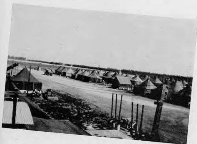
From atop of water tower, Mira Loma Street is viewed
