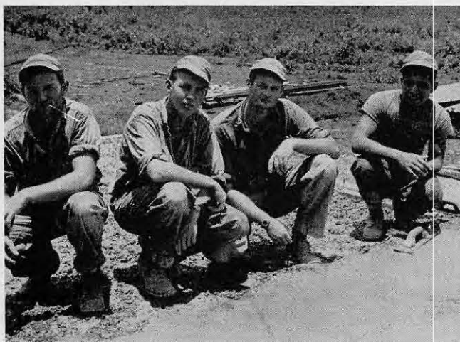
Crew poured foundation for ISCOM beauty salon
