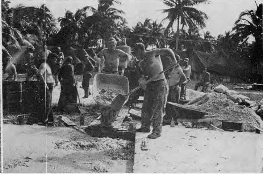
while cement crews constructed own forms, started pouring
