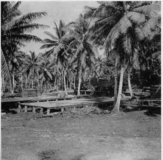
in Ninth area as tent platform foundations
