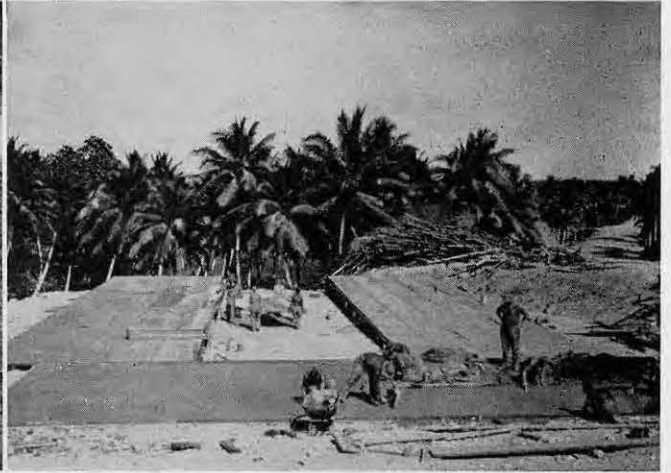
erected storage quonsets and built galleys for
