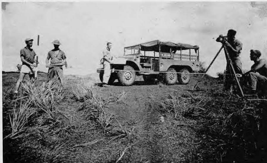
and battalion surveying crews started shooting the base lines
