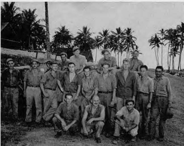
Interior electricians under CPO's Arp, Polye
