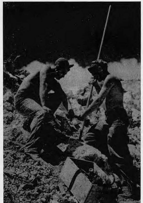
Herry Vorias and Al Failing tamp hole
