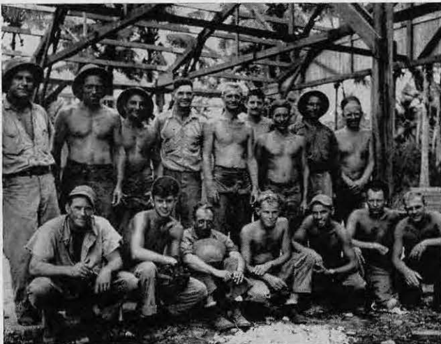
Chief Cox in charge of this Company A rigging gang
