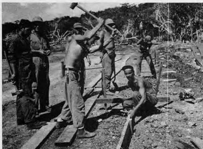
Forms for one of 574 concrete slabs is built
