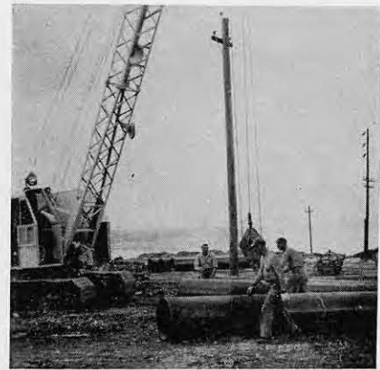
24-inch water line laid by Company A
