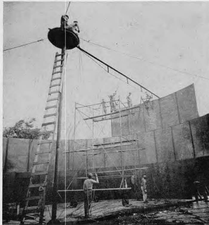
CB pulls a "Flagpole Kelly" at water storage tank
