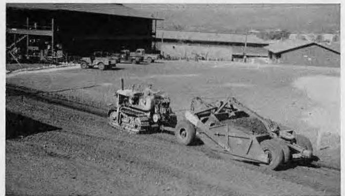
Pan moves in, spreading fill from an island pit
