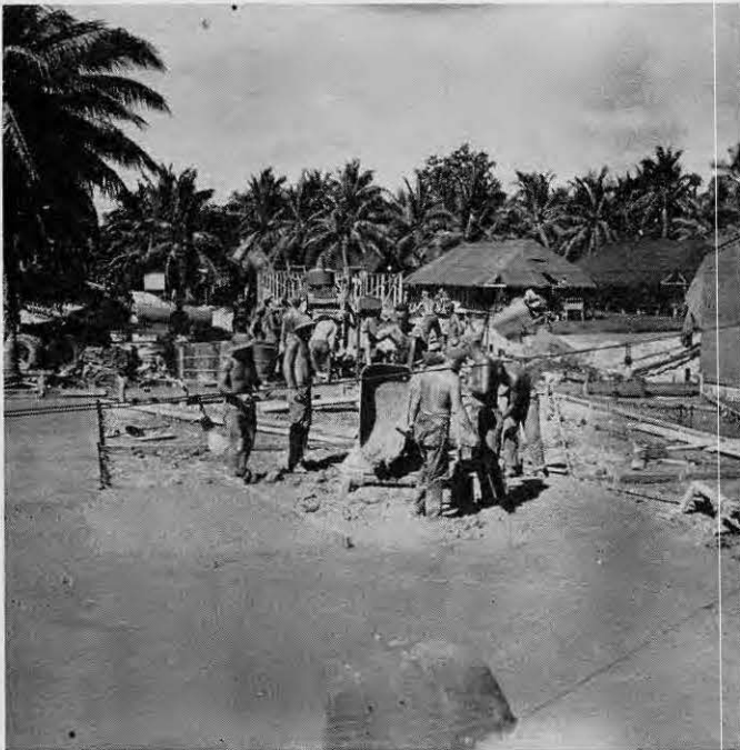
And finally after last load of concrete was in
