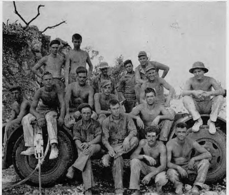
Jack-hammer and wagon-drill crews at quarry are shown
