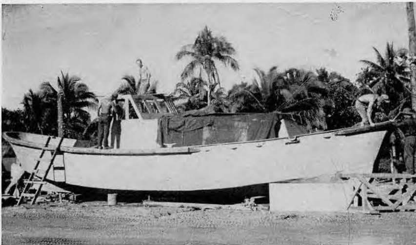
Odd sight was remodeled Jap landing craft in Trans. compound
