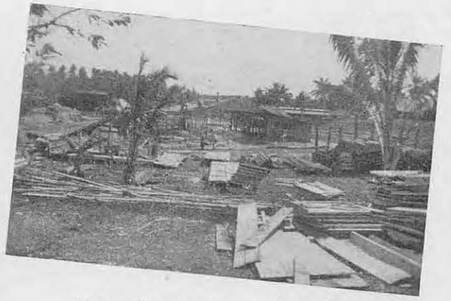
Compound construction sees shops going up
