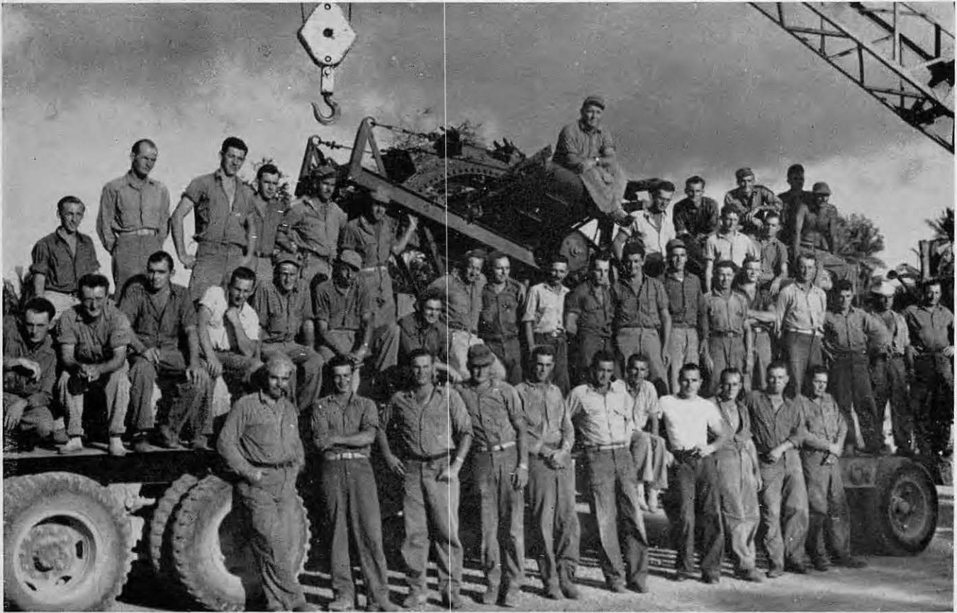
Led by Chief Jacob, 43 heavy equipment operators recorded by photog between shifts of 24-hour day
