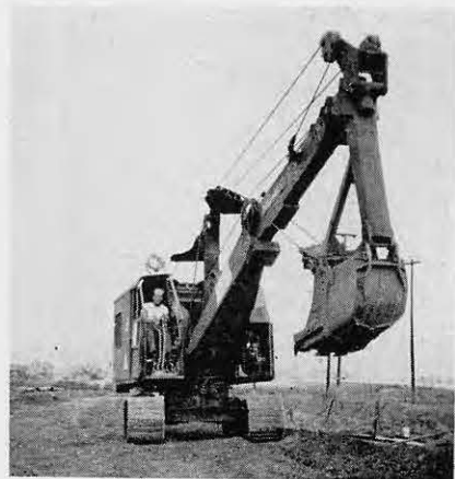
Digging ditch for water line
