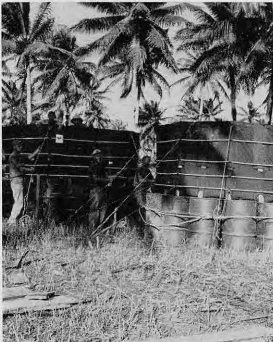
temporary water supply near the chow hall
