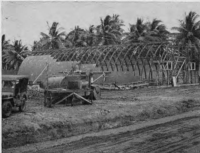
40x100 quonset, the GSK warehouse, is erected
