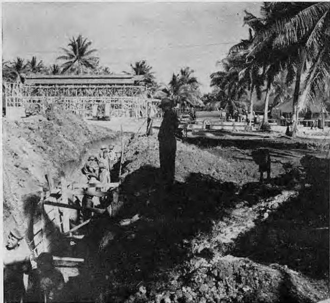
Drainage ditch cuts headquarters company area
