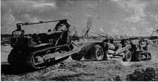
Two bulls, pan queezed in, break coral strata
