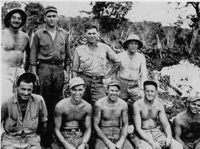
These two crews, directed by Chief Moore and
