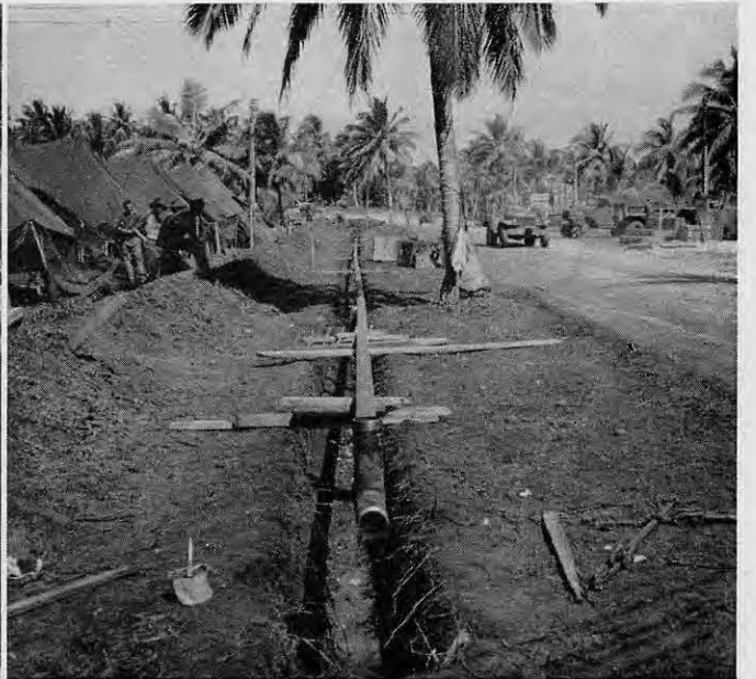
Main water line laid along main thoroughfare
