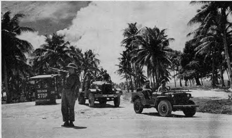
As sentry R. G. Hoffman stops traffic on highway, rig swings past
