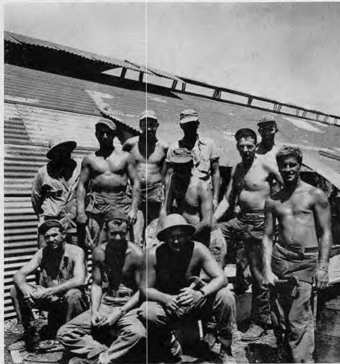
Ch. Matson's carpenters—Quonset hut facilities
