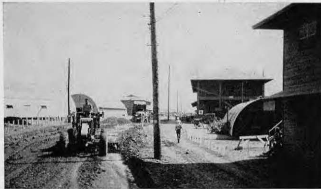
Patrol grading on main Ridge road near 103rd camp
