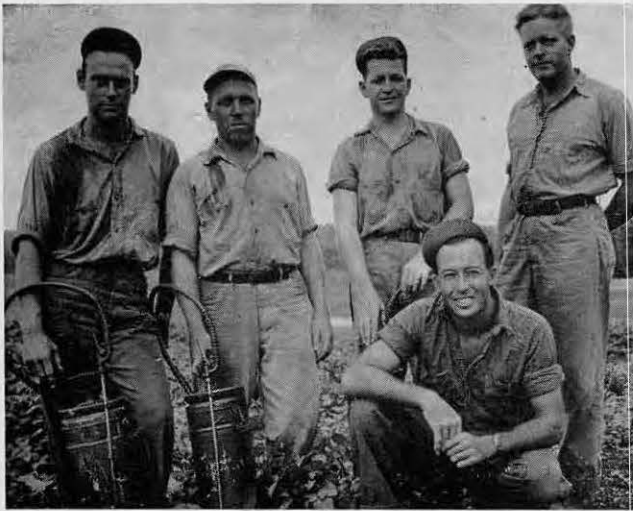
This was the first battalion sanitation crew
