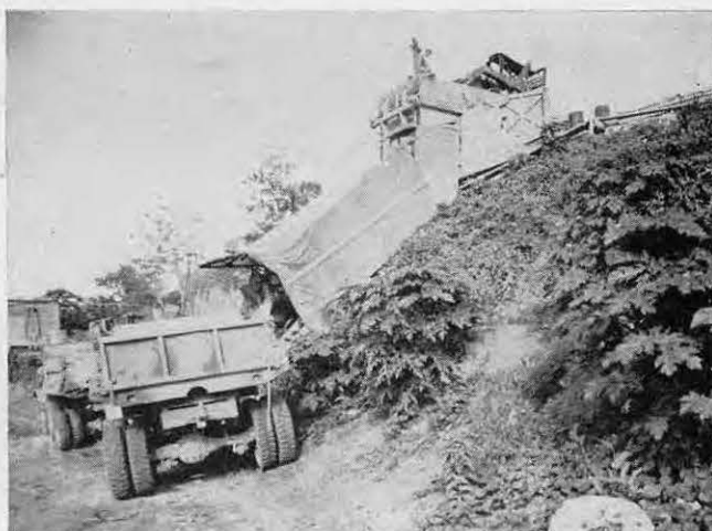
A cement plant was erected at the compound
