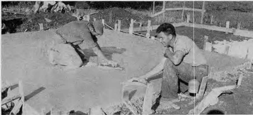
for new chow hall. Company A cement finishers took over shortly
