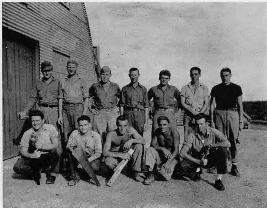
CPO Lincoln's crew of 11 set up the dairy's pasteurization unit
