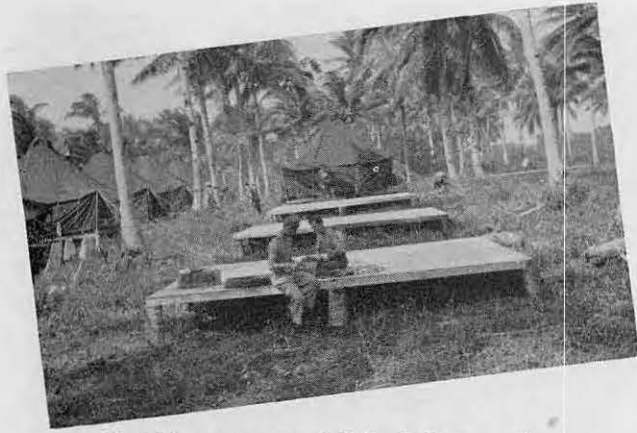
Electricians prepare tent lights in Company A
