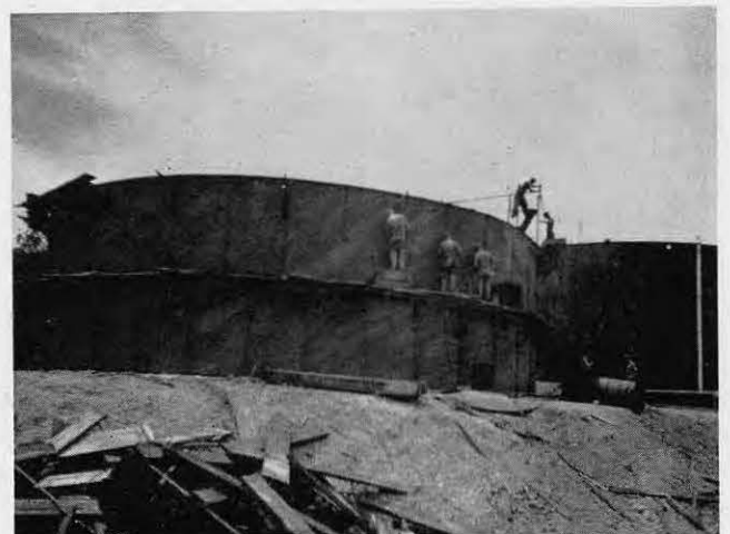
Dual water units, make an impressive picture
