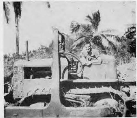
'Dozers cleared away the underbrush
