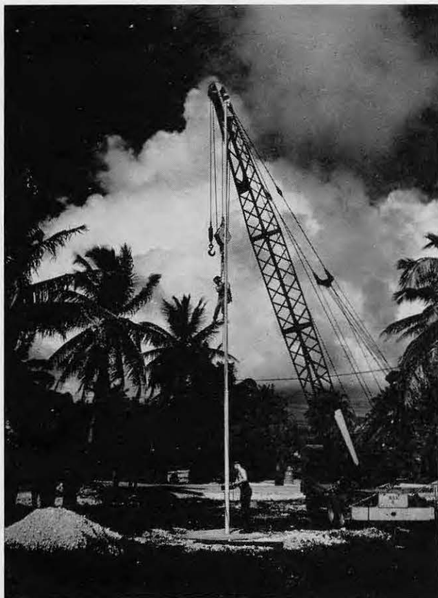
Crane raises flag pole in main area, topside
