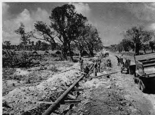
One string of 183,000 feet of pipe is laid
