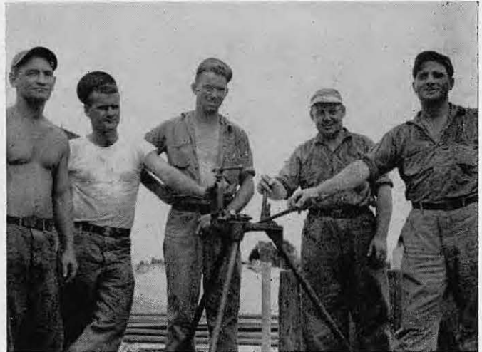
Company D shipfitter group headed by Chief Bello
