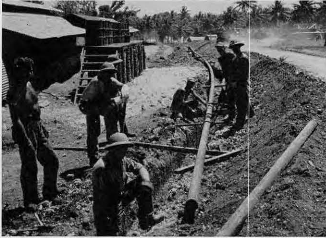
We put down pipe, laid out chow hall decking
