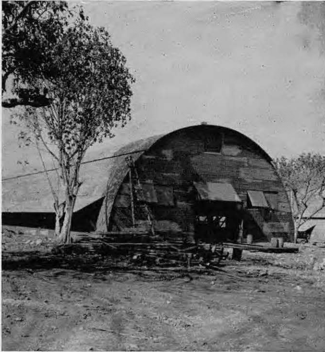
Work completed on the Sixth MarDiv front office
