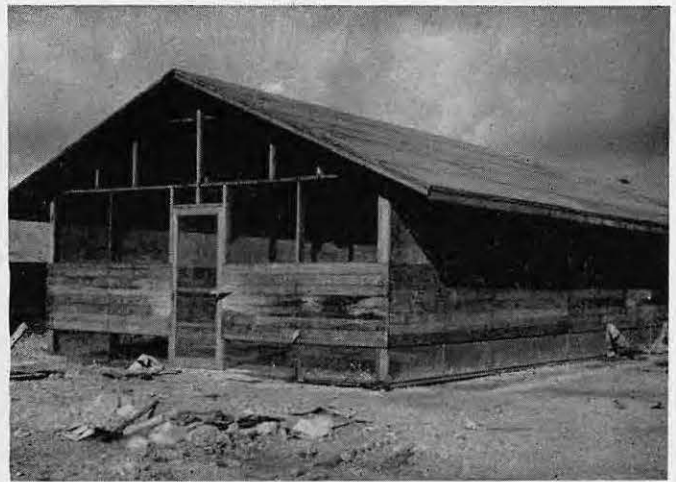
Completed prefabbed structure looks like this
