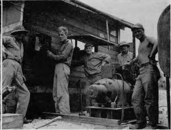
Electrical crew installs generator at crusher
