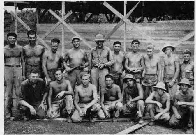
and Ludgate were Company A's erection gangs
