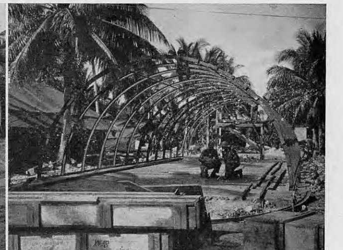
Construction goes on at "One Hung Low" laundry
