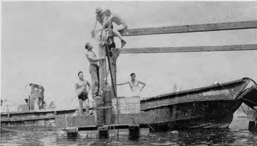
Last touch put to hoist apparatus—great moment is near
