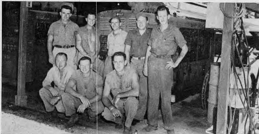
Generator men attended units that gave camp power and light
