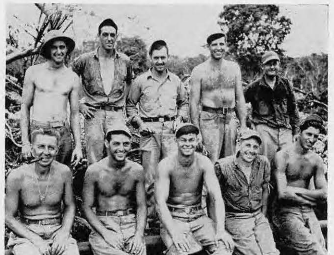
Weycker, laid heavy pipe lines over the camp
