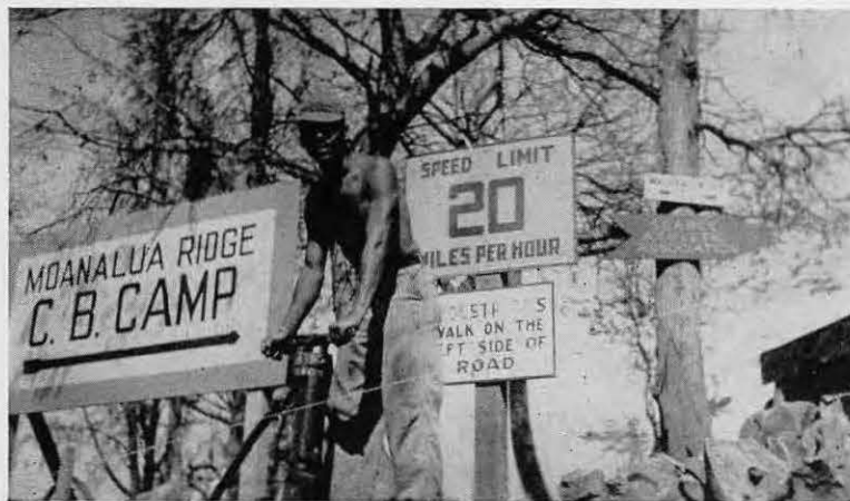
Lou Nunez wields hammer at main entrance to Ridge area
