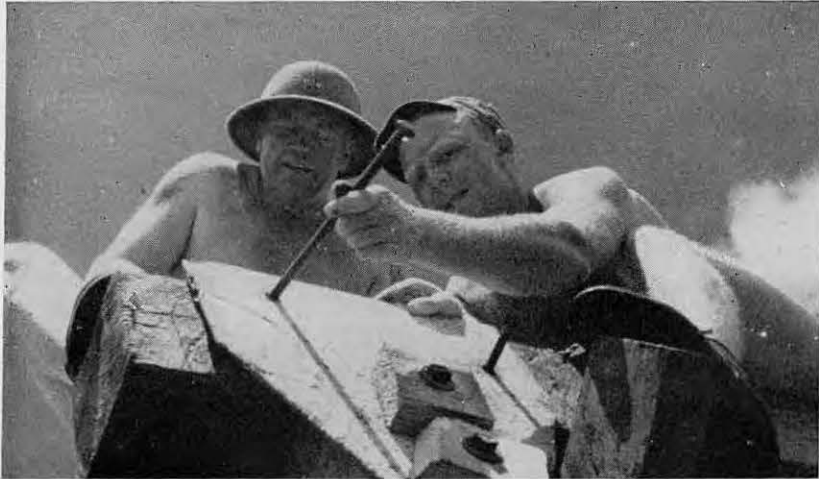
Chief Ness and Bert Streblov set driftpins on pontoon hoist
