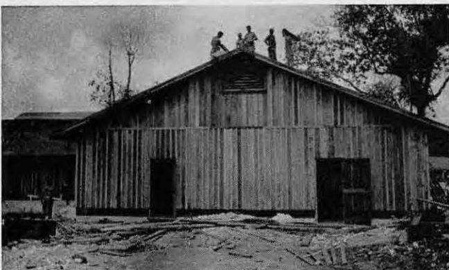
103rd roofmen near end of chow hall structure
