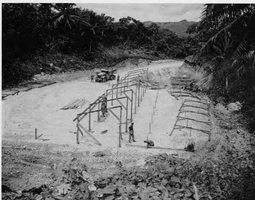
Battalion carpenters prepare shelters at Ammunition Dump No. 15
