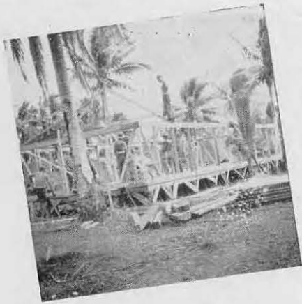
First work on camp sick-bay
