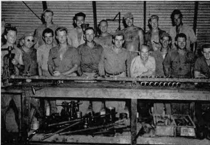
Ch. Fehmel's line gang of fitters and welders
