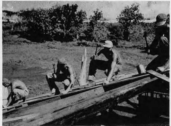
Carpenters lay roofing onto Sixth warehouse
