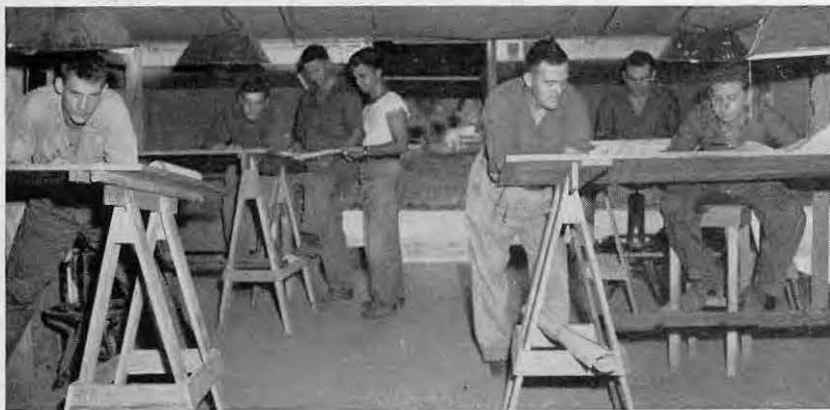
Then design engineers mapped the entire zone into 12 areas
