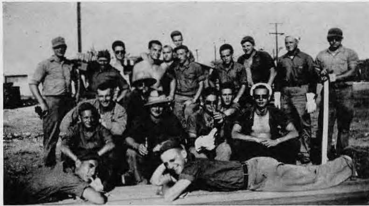
Lumber yard crew was composed mainly of 103rd band members
