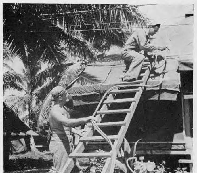
Waterproofing done by Joe Lopez and Vern Jones
